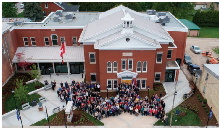
▲ After extensive renovations, the Blyth Memorial Community Hall was reopened on May 19, 2017. Photo Rob Boyce, 2017
