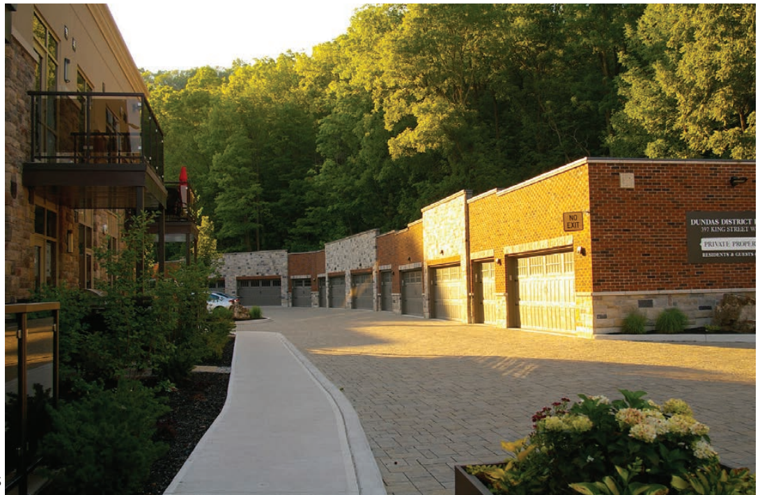
Rear façade of Dundas District Lofts and the north garage structure, incorporating the crash wall. Photo Ann Gillespie, 2016
