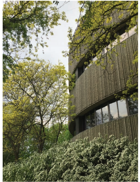
The textured concrete walls support Moriyama’s vision that everything be tactile. Photo Ontario Science Centre, 2016
