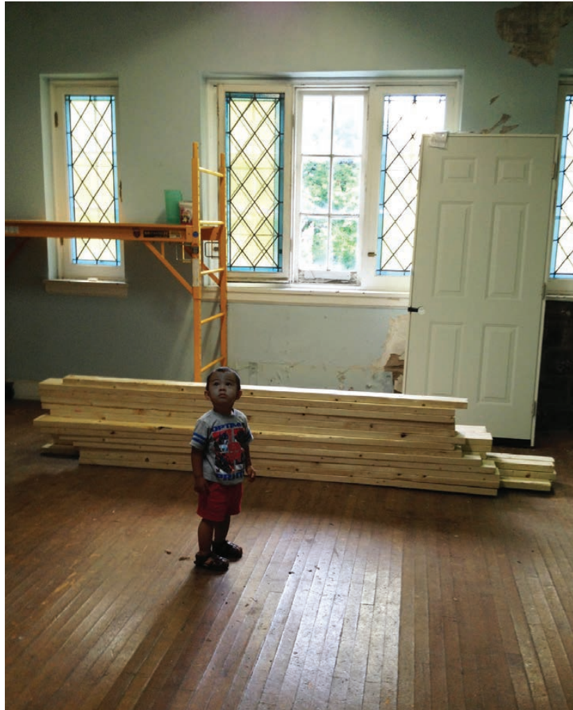
During renovations inside the Parish Hall. Photo Bonita Slunder, 2014
