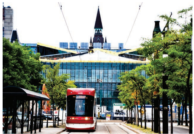
View of construction from the north. Photo Richard Longley, 2016
