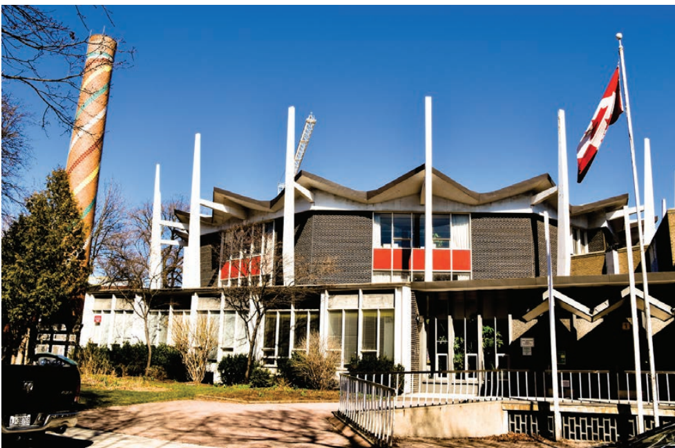
Lord Lansdowne Public School at 33 Robert Street in Toronto. Photo Richard Longley, 2016
