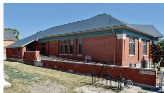
▲ The new ramped entrance creates a brick base for the original building. Photo Dan Schneider, 2018
