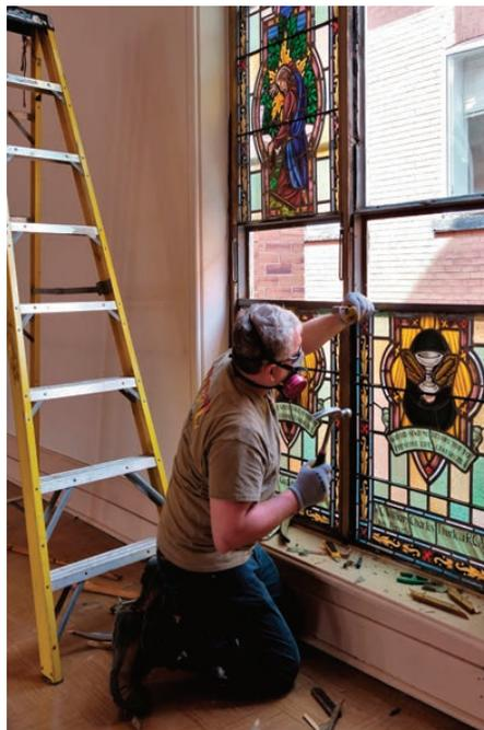
▲ Wearing a respirator and protective gloves, Adam Frazee of Sunrise Stained Glass is using a hammer and chisel to free a section of one of the larger 1950s Luxfer windows.
