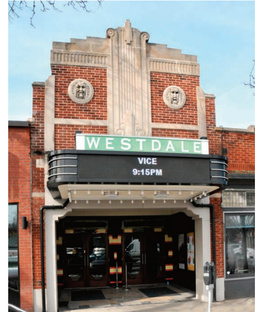
The restored Westdale Theatre reopened in February. Photo Shannon Kyles, 2019
