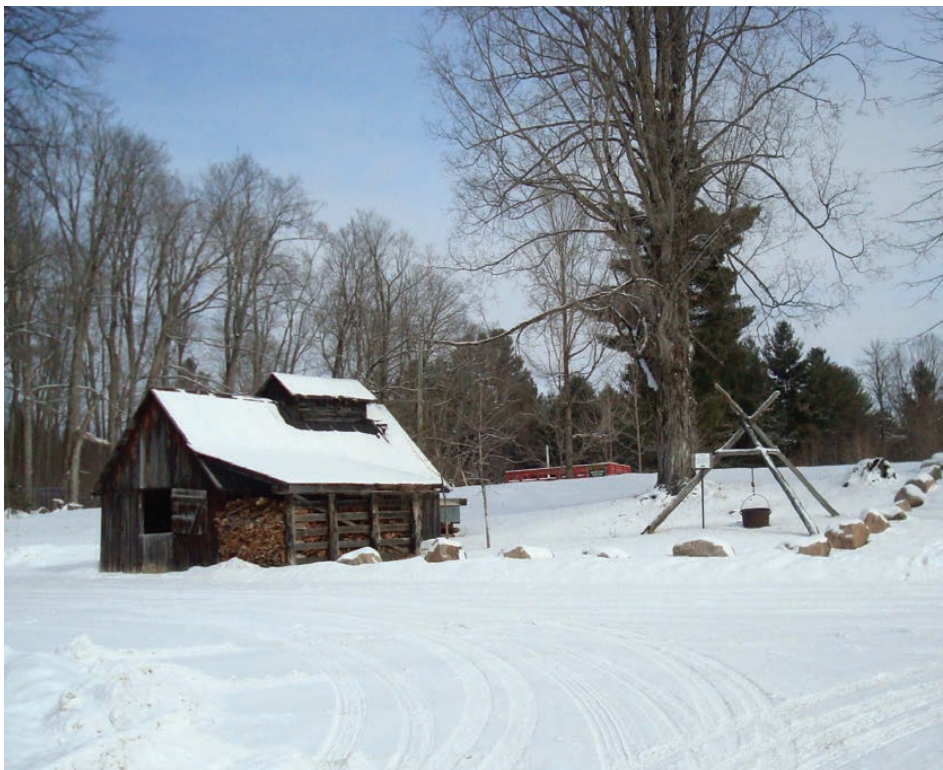
Vernon Wheeler preserved the sugar shack built by the Robinsons on the property in 1936. Photo Liz Lundell
