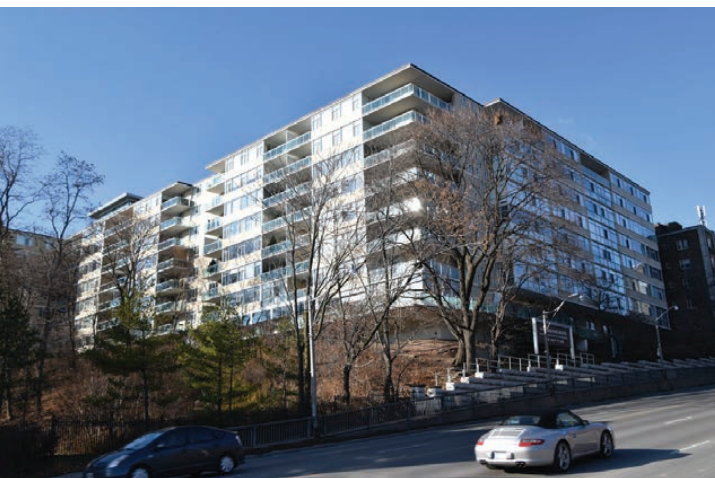
Benvenuto Place, Avenue Road, Toronto, 2016. Photo Richard Longley
