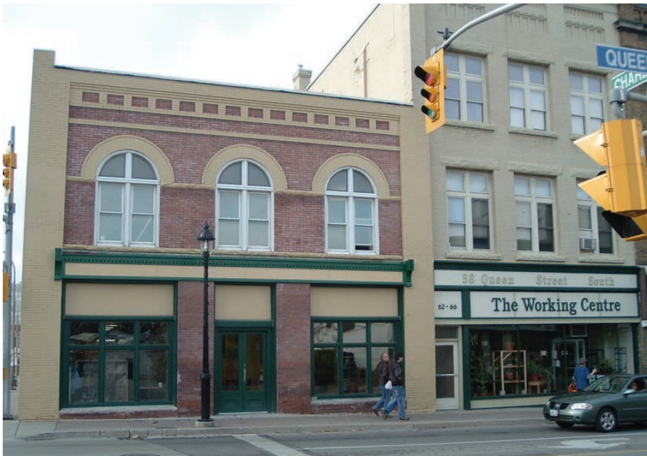
The restored exterior of 66 Queen Street South, Kitchener, 2006. Photo Joe Mancini
